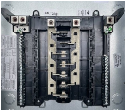
Figure A - Typical Main-Lug-Only Electrical Panel Busing
